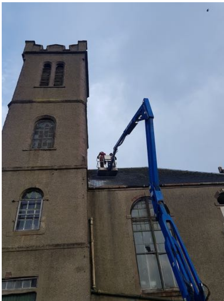
ARA inspection of east face of tower
