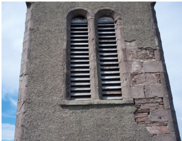
-2105281226 east view of the tower belfry level © A. P. Rodger 2022
