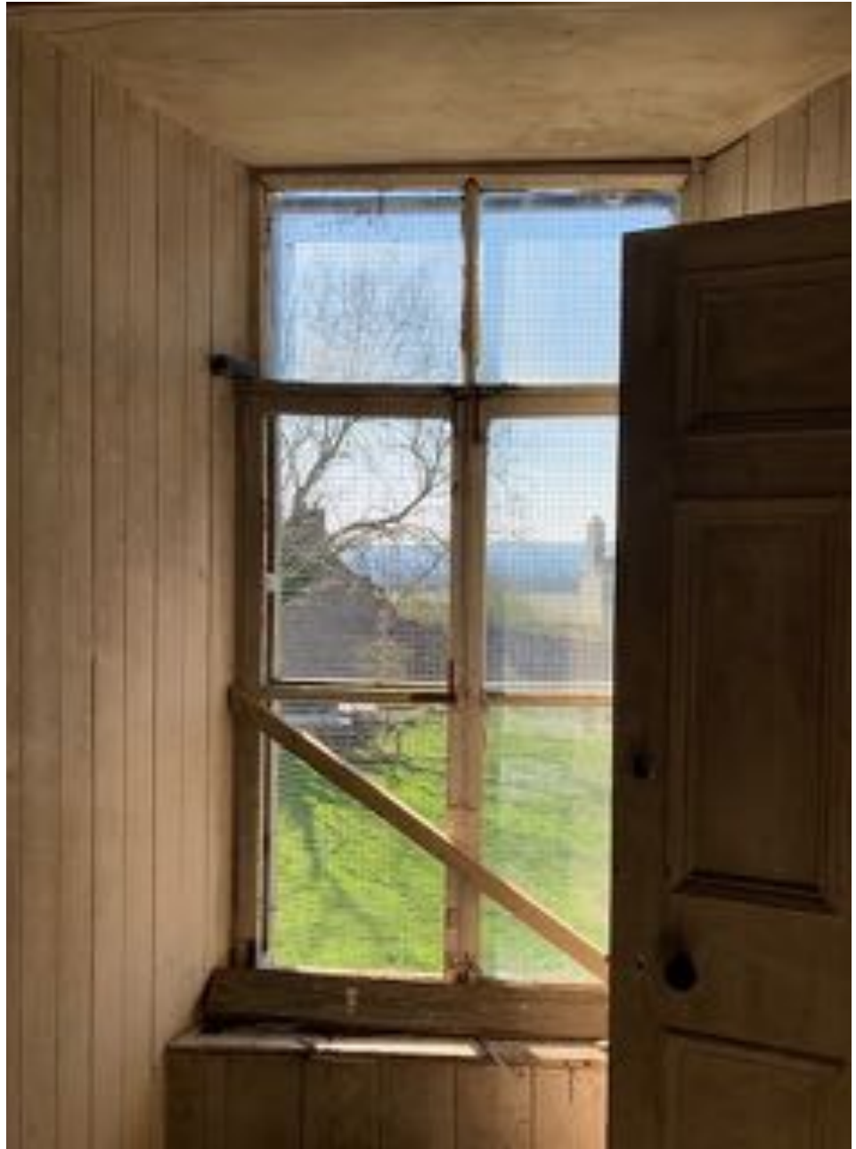
GW06 with secondary glazing on lower portion. © A. P. Rodger 2021
