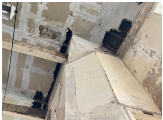
View of the tower corner cantilever from main space
