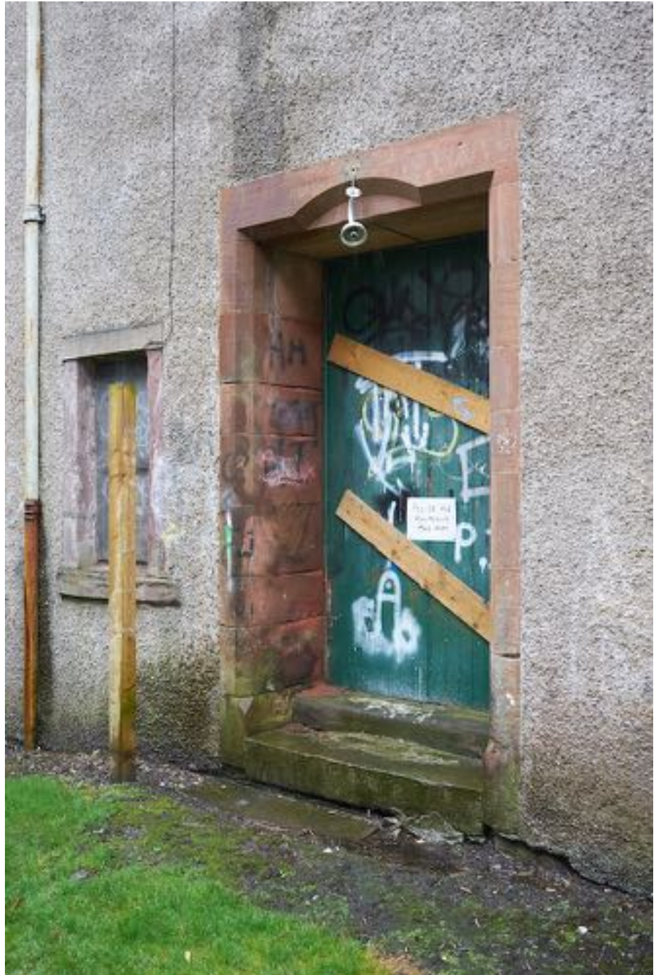
GD04 + GW10 - North doorway with lighter coloured sandstone reveal © A. P. Rodger 2020
