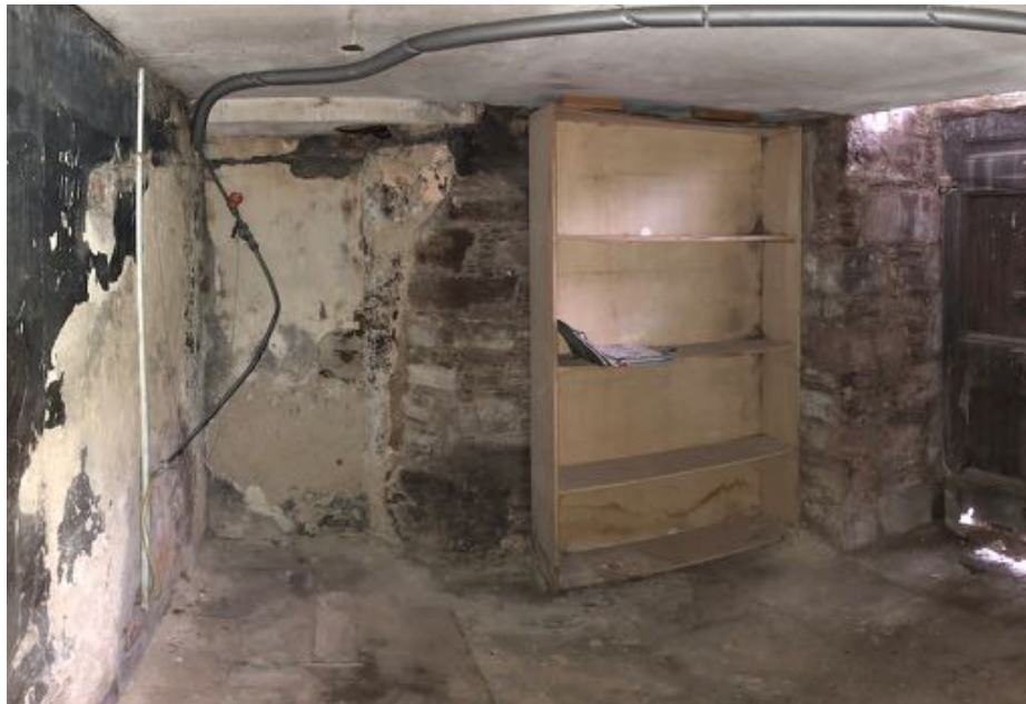
View of east side of the tower, level 1 © Andrew Rodger 2021
