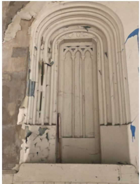
Doorway from former pulpit location to tower
