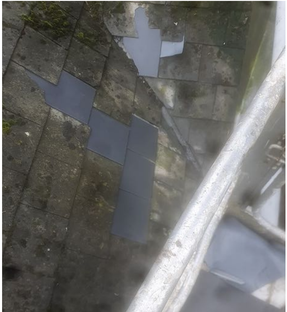
West side of saddle roof valley as repaired © Ryan Scott 2022
